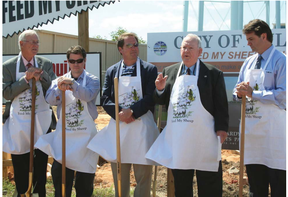
Celebrating the groundbreaking for Feed My Sheep's new facility are (left to right) board member Ted Hearn; Johnny Olsen, Guild Hardy Architects; Gordon Myrick, H. Gordon Myrick, Inc.; Joe Steinwinder, chairman of the board; and Gulfport Mayor Brent Warr.
